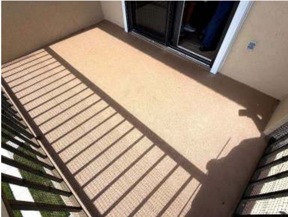
View of typical balcony
