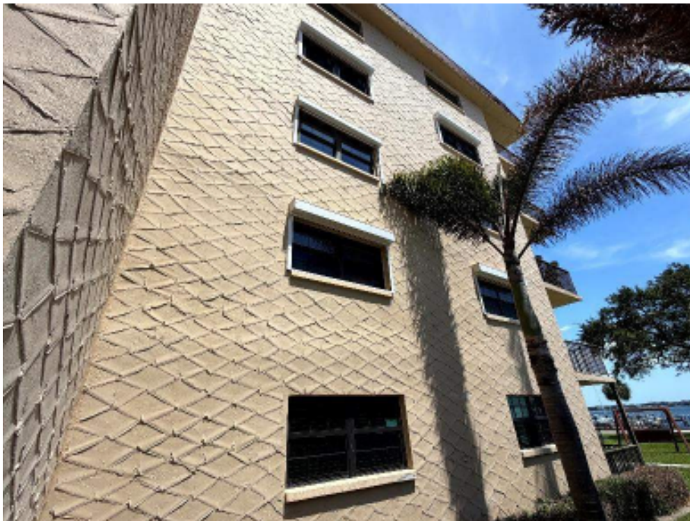
View of south elevation
