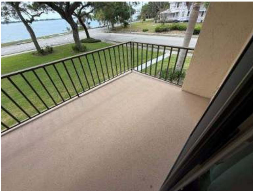
View of typical balcony
