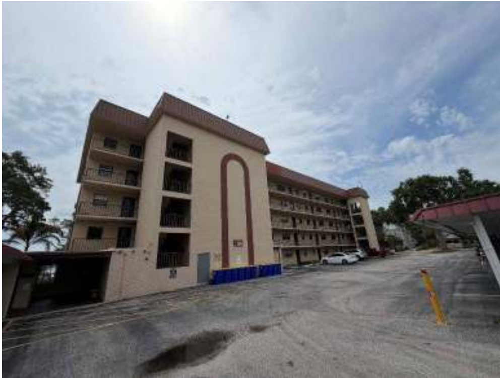
View of west elevation
