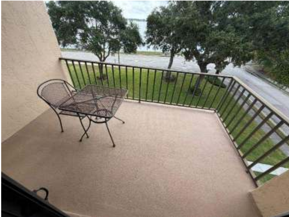
View of typical balcony
