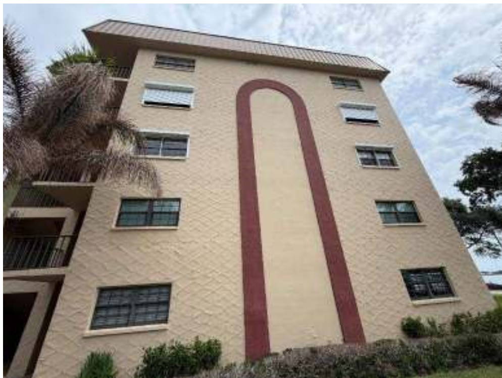
View of south elevation
