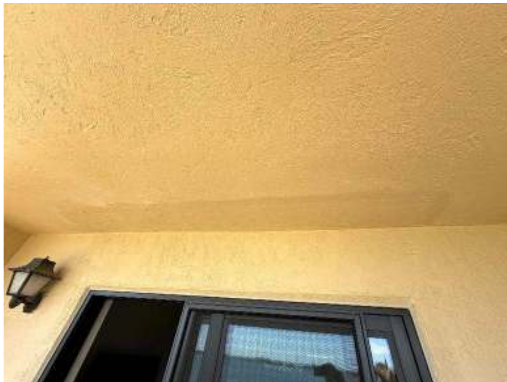
View of previous ceiling repair
