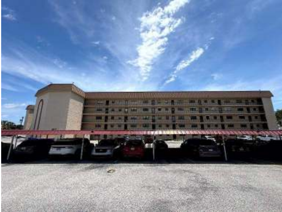
View of west elevation
