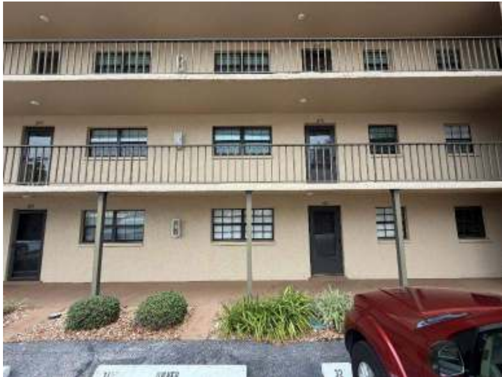
View of west elevation
