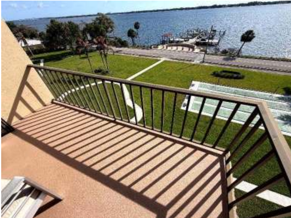
View typical balcony
